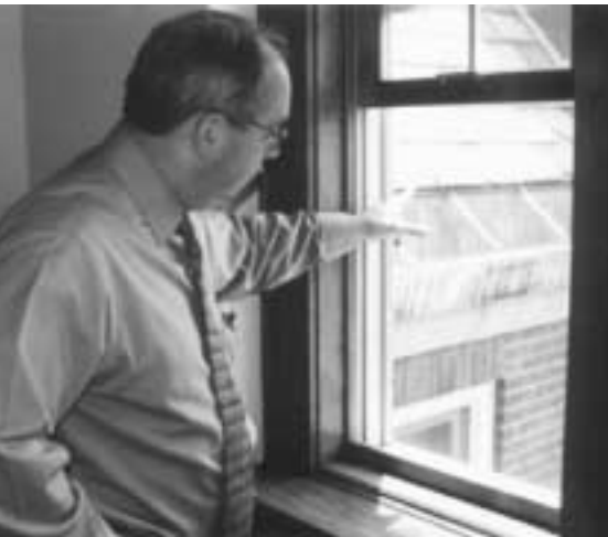
Building Administrator John Duncan points out an area of chapel roof gutter than has been re-lined to prevent water damage.
